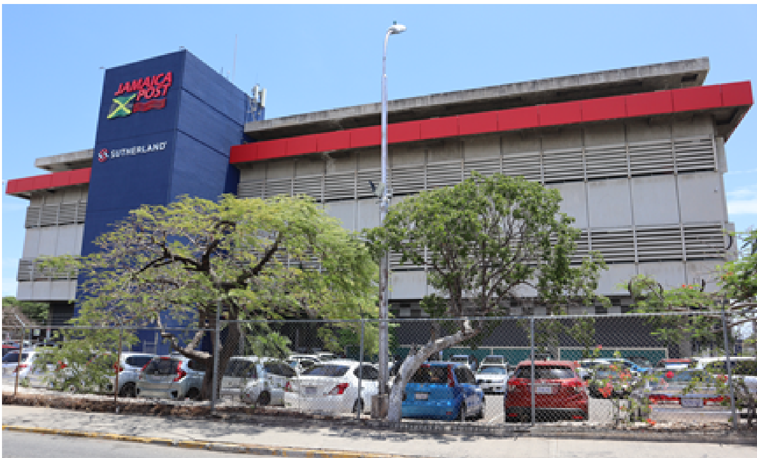
Post and Telecommunications Department (Jamaica Post), 6-10 South Camp Road, Kingston boasts brand new signage, with sections of the exterior of the building that have been freshly repainted.
